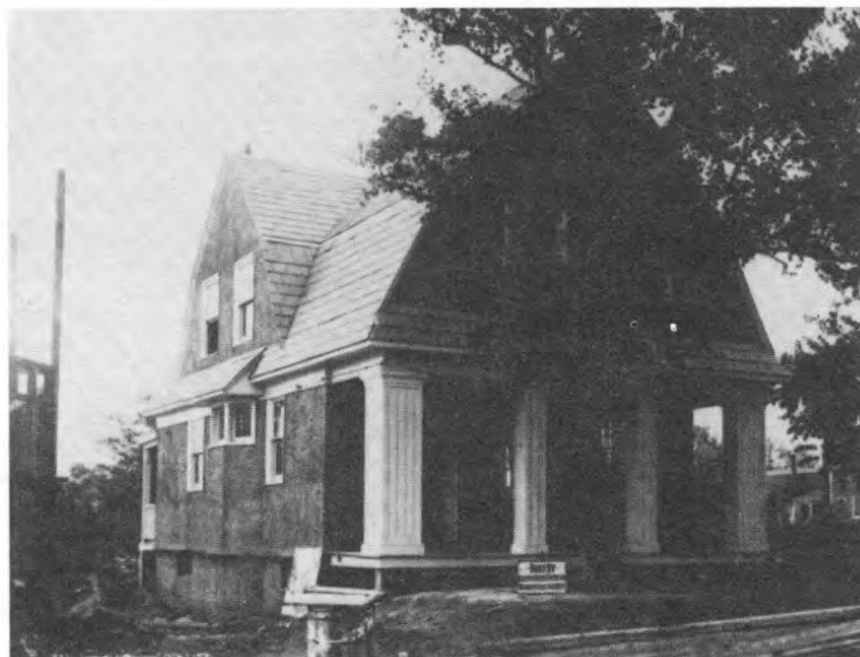
Figure 5. The residence of A.M. Strong at 5410 Young Street (formerly 76 East Young Street), Halifax, had a unique design by Ross and Macdonald. (PANS, negative N-7040)
